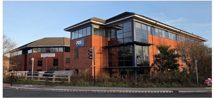
PDS Infrastructure Systems
